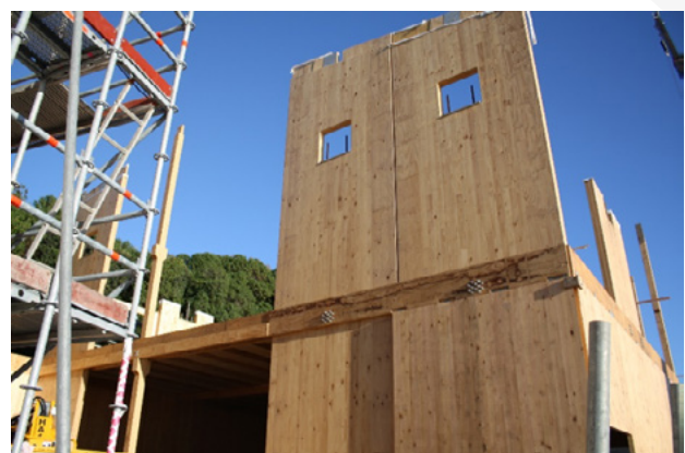
KDC rocking shear wall
