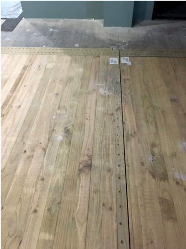
Repaired Floor Panels
