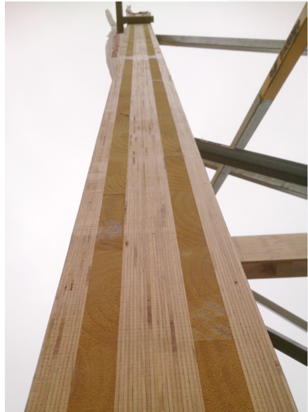
Composite LVL/XLam rocking shear wall
