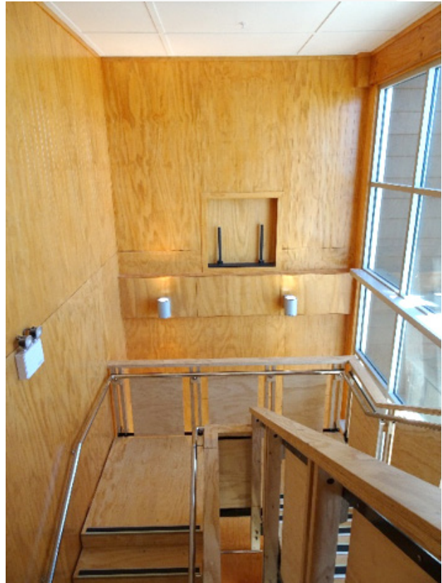
Rocking shear walls show little sign of damage
